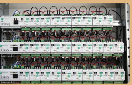
TOZD is power source module for TO5Dp and TO3Dp. Includes two separate circuits 24 VDC, first is for feeding of control circuits of TO modules, second is used as power for binary remote control, when used. TOZD have LOCAL / REMOTE switch with signalization and voltage loss contacts.
