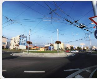
For roundabout solution is suitable use of double switch point controlled by VETRA system with fully automatic operation.
