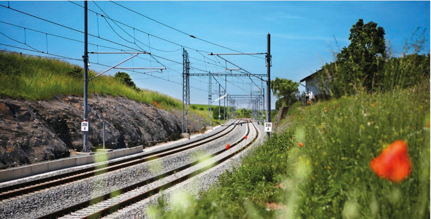
Elektroline provides complete production and installation of modern catenary (rail overhead) system ARCAS-EL, which is suitable for all traction voltage systems. Designed for railways track with speed up to 250 km/h.
