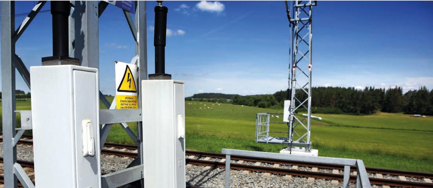
Elektroline manufactures and installs motor drives of traction disconnectors that are designed for use with all types of sectional disconnectors, power disconnectors, earthing switches.
