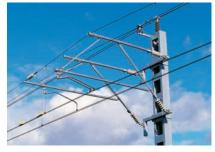
Cross arms for double support structures are equipped with the same swivel joint as the single support structure.
