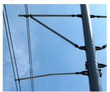
For maintenance work or where clearances are not clearly defined by the design, the lateral support offers the advantage that it can easily be cut to the required length on site.
