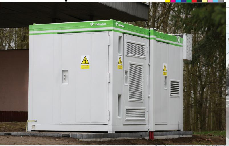
This station is located where the OCS does not meet the energy required for trolleybuses. Typically, these areas are located far from power substations as the longdistance resistance of the wires causes a voltage drop. Instillation of the station occurs when the catenary is powered by only one converter station, typically during reconstruction. The buffer station can compensate well for a lack of tension in the system.
