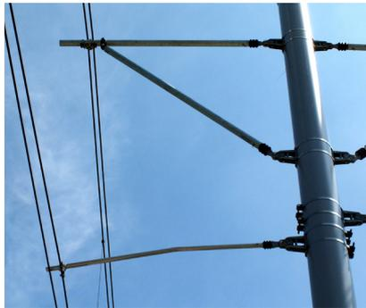
For maintenance work or where clearances are not clearly defined by the design, the lateral support offers the advantage that it can easily be cut to the required length on site.
