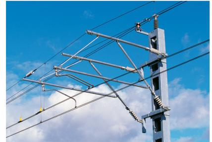
Cross arms for double support structures are equipped with the same swivel joint as the single support structure.
