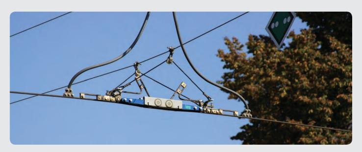
A special construction of our section insulators allows a silent and fast passage of the pantograph. Our section insulators are designed in such a way to safely interrupt both common equalizing currents and contingent short-circuit currents.
