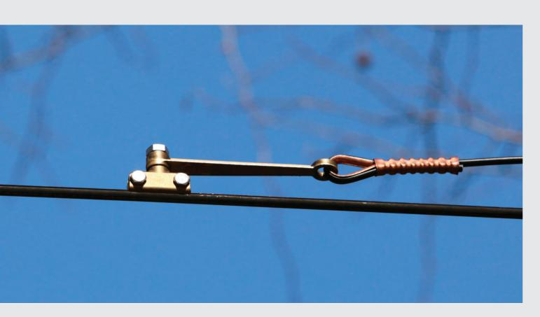
Elektroline company provides wide assortment of self made contact wire clamps whose parts are manufactured form various kind of material, eg. copper alloy, stainless steel, and others.
