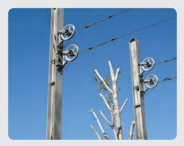
A latch on the compensation wheel prevents the weights from falling to the ground during OCL accidents. Wheel compensation transmission ratio is 1:3.
