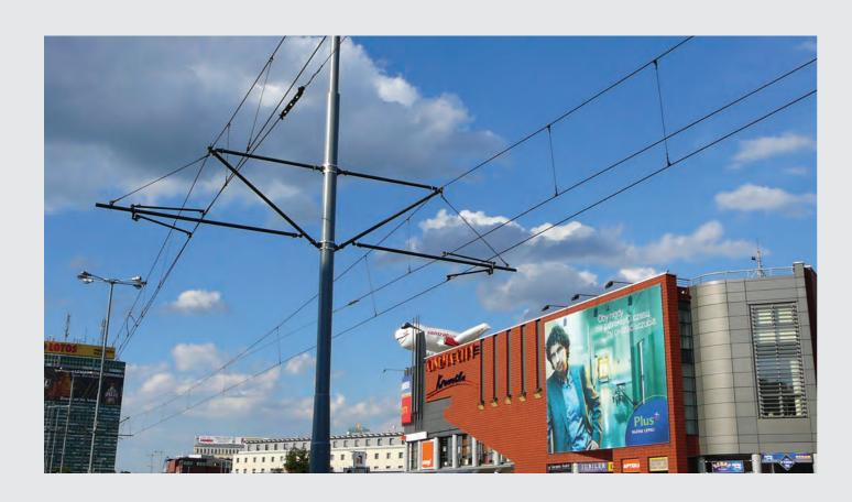
Catenary system is usually used on the tracks where higher operating speed of vehicles (over 90 km/h) is required.
