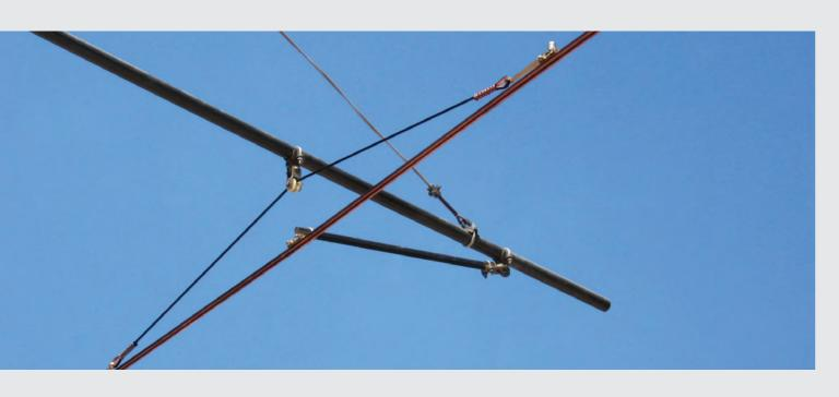
The overhead contact line with suspension of delta type in combination with temperature compensation represents a modern type of overhead contact system. This type of contact line satisfies high requirements imposed on the tram operation.
