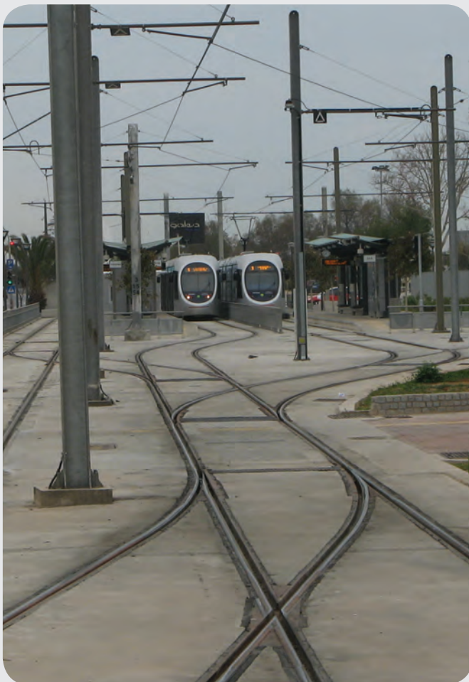
Elektroline signaling system in Athens, Greece
