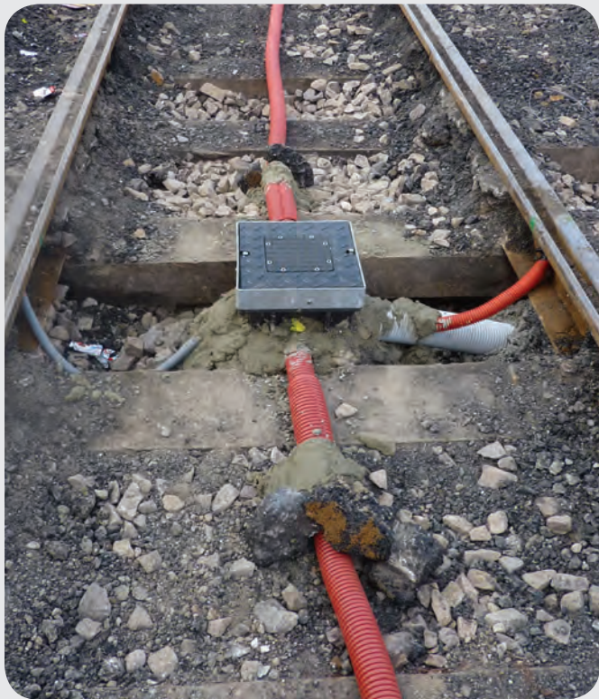
Connecting a track circuit in the tracks
