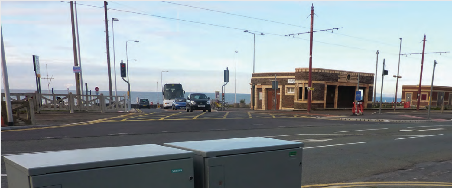
Elektroline tram priority system (United Kingdom)
