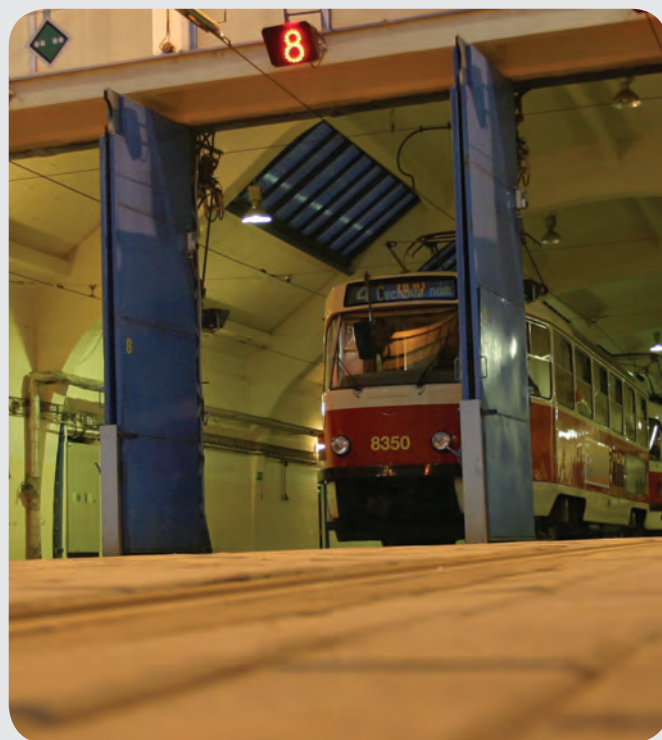
Fully-automatic depot control system (Prague)
