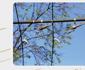
Curve clamps fixed on GRP cantilever
