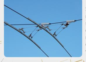
Supporting net made from KEVLAR synthetic ropes decline undesirable noise which is characteristic for vehicle's moving.
