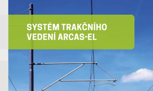
Elektroline provides complete production and installation of modern catenary (rail overhead) system ARCAS-EL, which is suitable for all traction voltage systems. Designed for railways track with speed up to 250 km/h.
